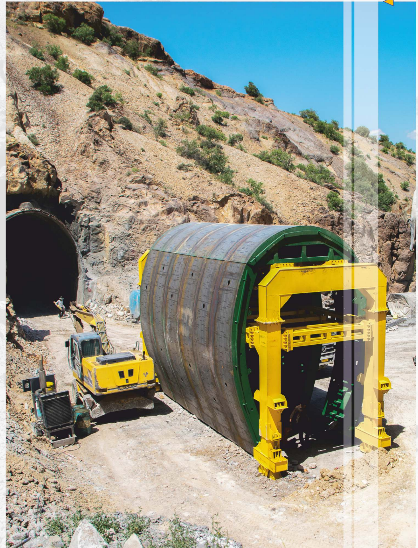
Tunnel on the Mianeh – Ardebil Railway – Part 3B
