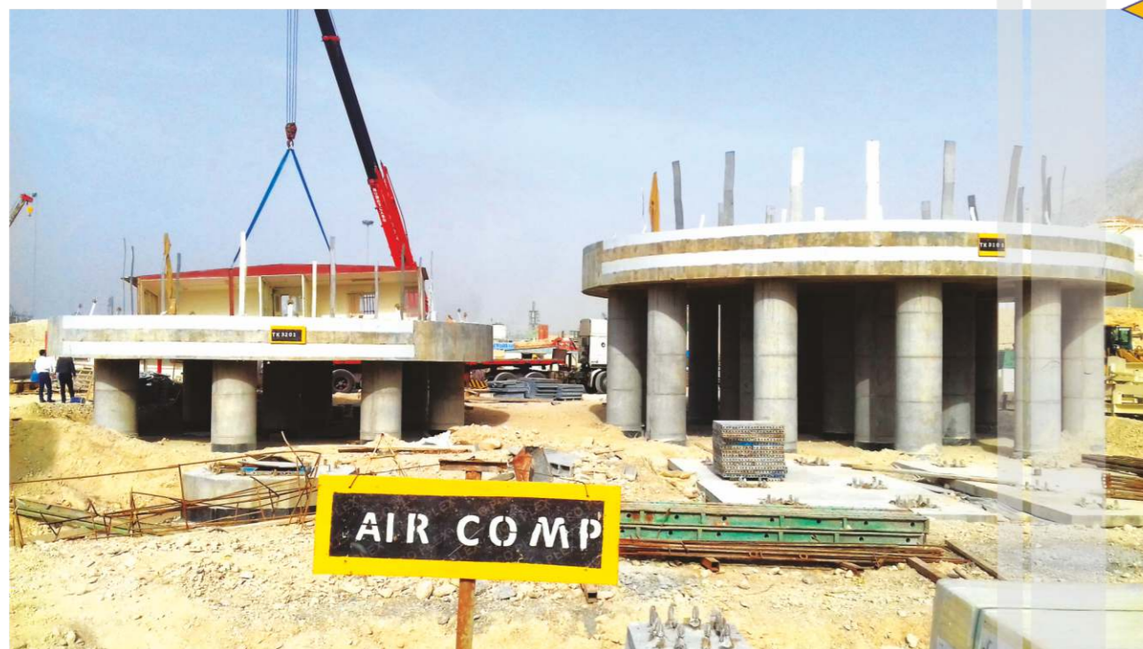
Air Compressor Foundations of ASU Project
