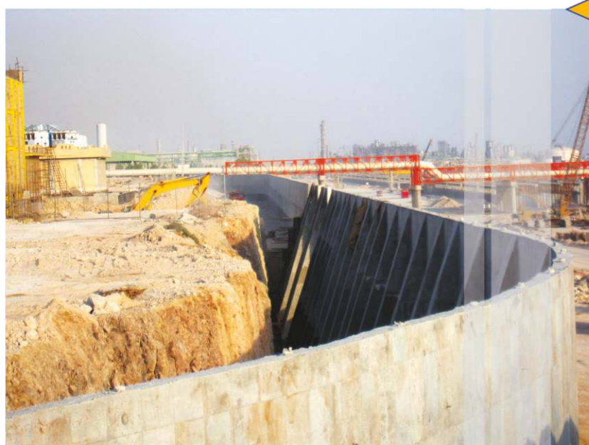
Construction of Retaining Wall around Morvarid & Kavian Petrochemical Complexes in Asaluyeh
