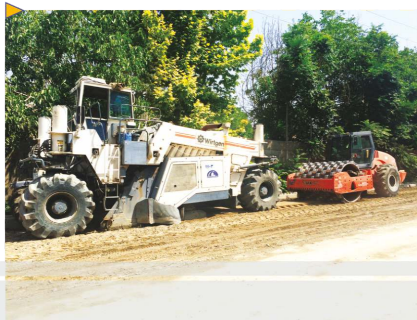
Asphalt Cutting, Stabilization & Pavement of Payam St. in Lavasan Cit
