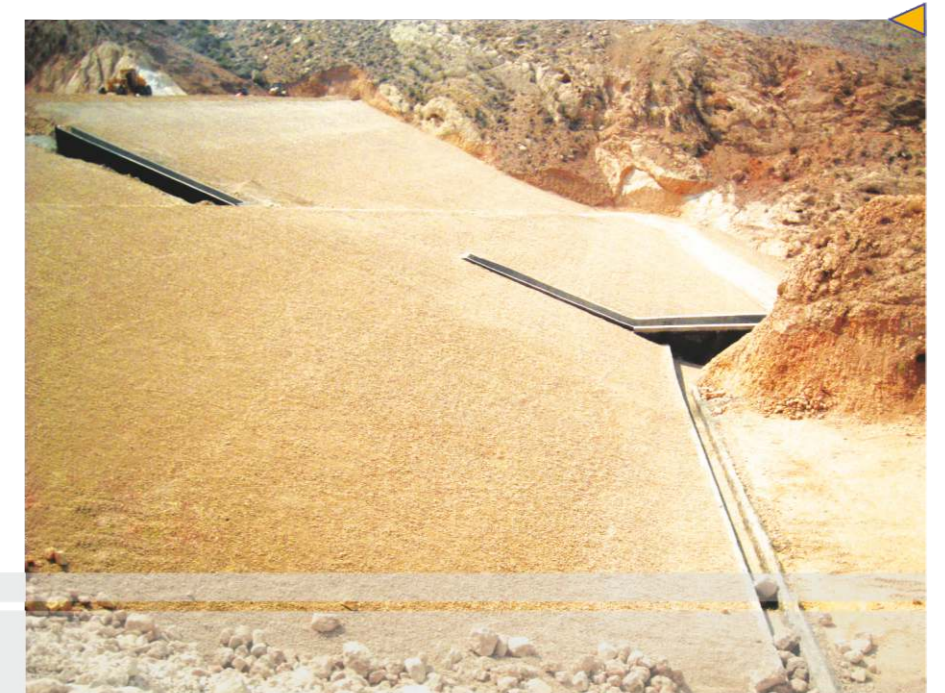
Construction of S3 Detention Dam in Asaluyeh
