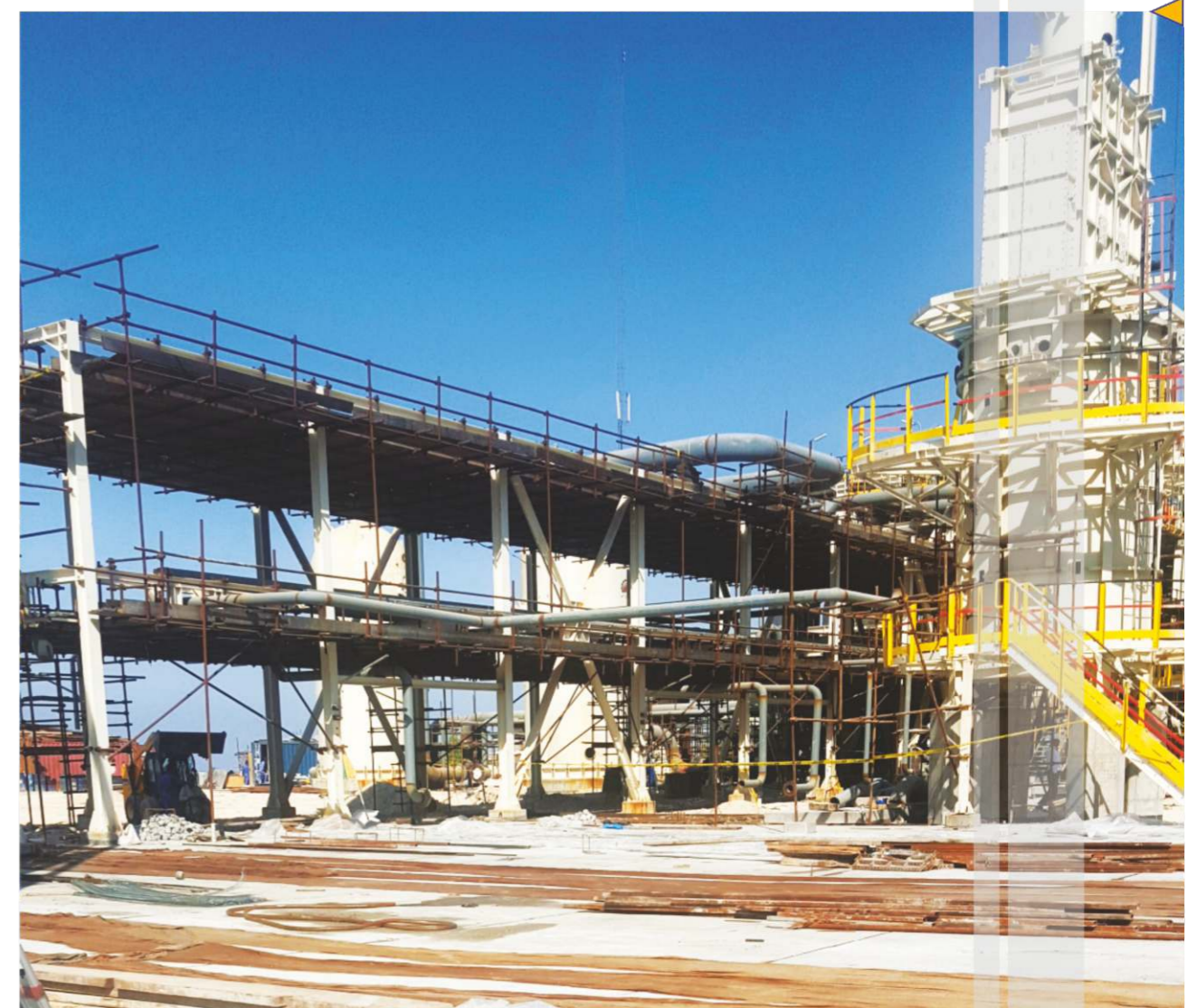
Paving of Sweetening Unit of Boushehr Petrochemical Complex in Asaluyeh
