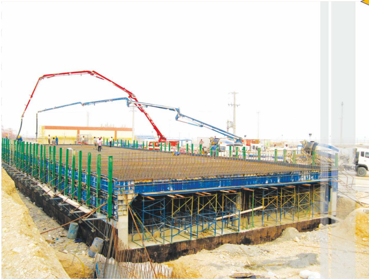
Construction of Instalation Culvert & Sleepers in Kavian Petrochemical Complex in Asaluyeh
