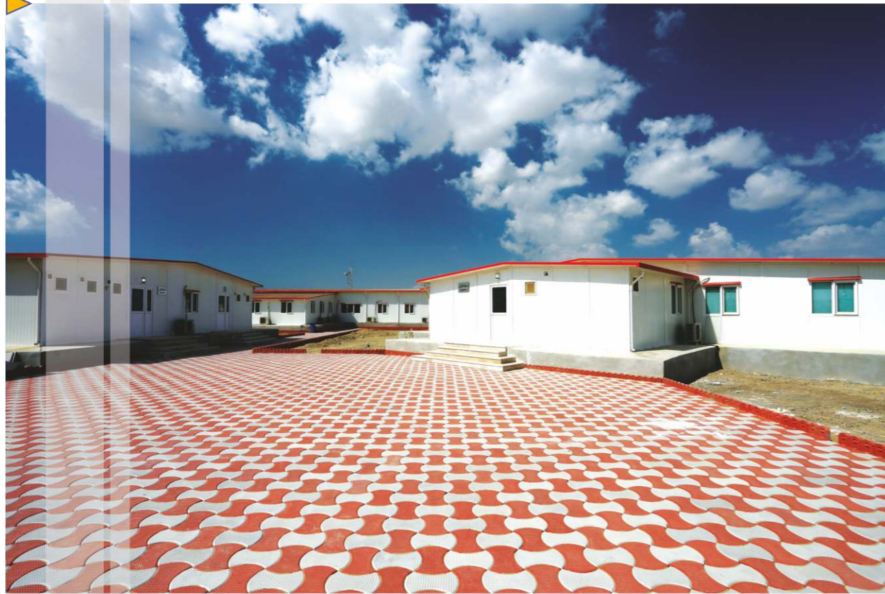
Counstruction of Administrative Building Site of Makran Petrochemical Complex in Chabahar
