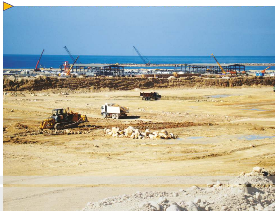
Trenching & Preparation of Second Phase of Asaluyeh Petrochemical Complex
