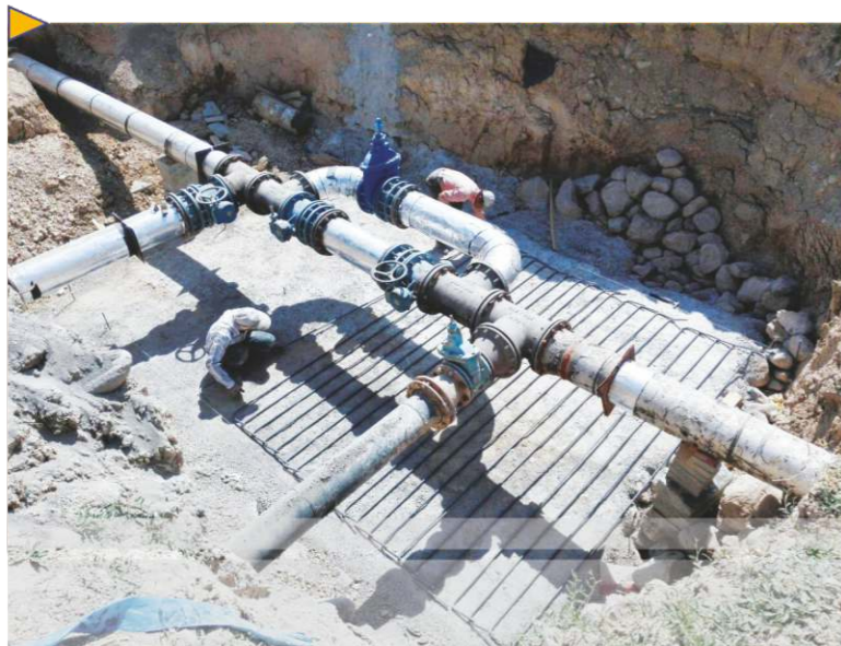
Construction of Water Conveyance Network to the Zones of Ardebil City
