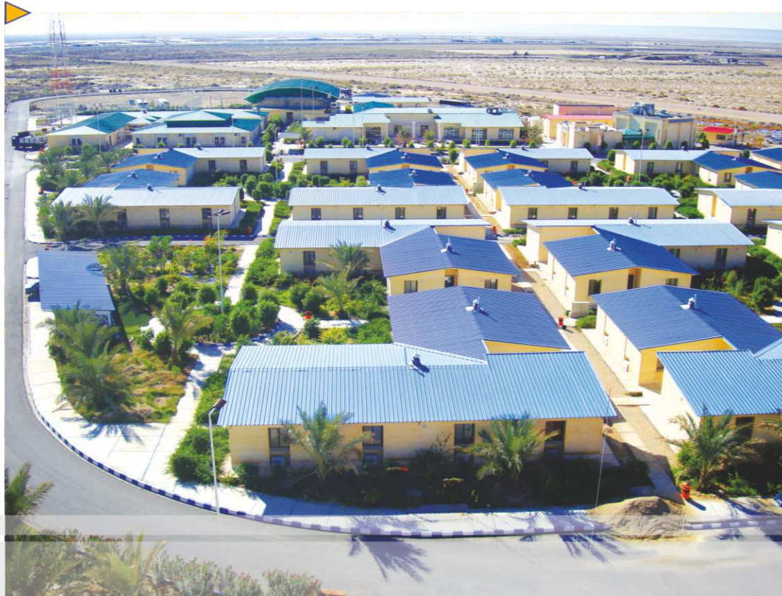
Design, Procurement & Construction of Bidkhoon Residential Complex in Asaluyeh
