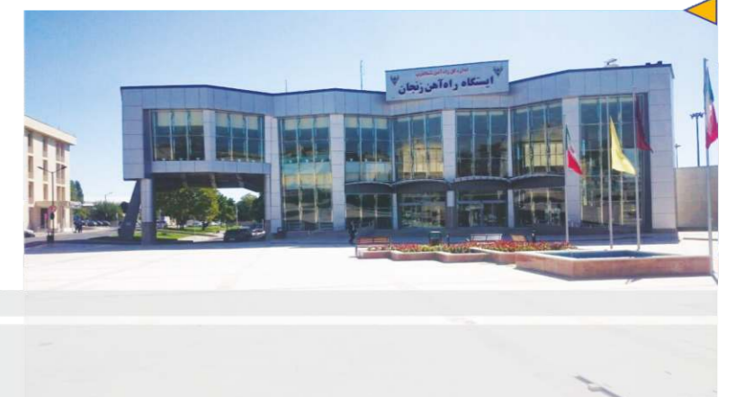
Building Construction of Zanjaan Railway Station
