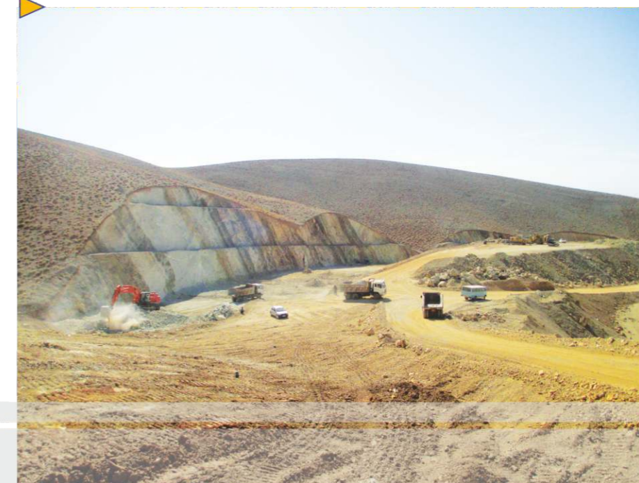
Construction of West Ringway of Damavand City
