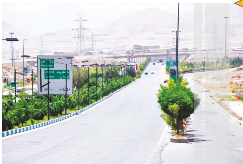
Earthworks & Asphalt Implementation of Parts of Pardis New City (Phases 1,2,3)
