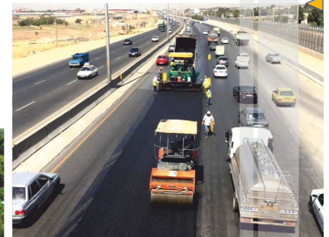
Hot Thin-Layer Polymer Modified Asphalt of Karaj – Qazvin Highway (Karaj – Hashtgerd)
